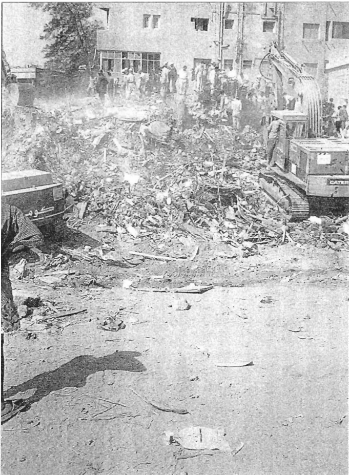
Left: Remains of a 14 storey reinforced concrete building that collapsed. Teams from Italy, Germany and France helped with the rescue operations.
